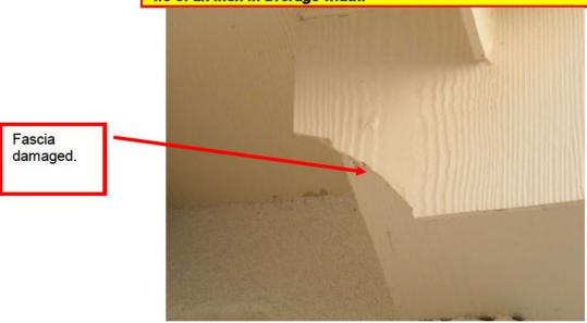
The soffit and fascia above the hinge side of the courtyard gate has not been caulked or painted as required by the materials manufacturer, IRC 102.4 and 703.1, and 703.10.1. From the builder's warranty:
