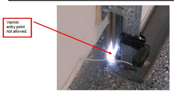
Rodents destroy insulation, electrical wiring, plumbing, and other structural components of buildings (Fig. 1). Insulation damage alone may amount to a loss of several thousand dollars in only a few years. Energy loss from damaged buildings results in added annual costs. Rodent-induced fires from damaged electrical wiring or nest building in electrical panels cause loss of property and threaten human safety.
