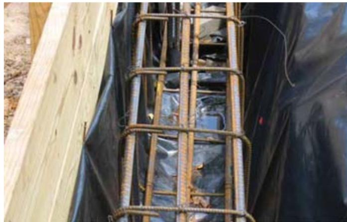
Photo 2. Close up. Vapor barriers create isolation between the concrete and the earth. These are not suitable for use as concrete-encased electrodes.
