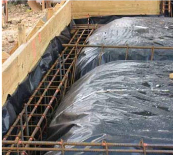
Photo 1. Vapor barriers create isolation between the concrete and the earth. These are not suitable for use as concrete-encased grounding electrodes. (Photo courtesy of Robert Jones, IEC)
