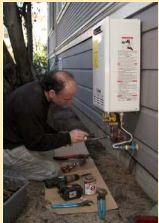
**Figure 6.** The author gained valuable floor space in this house (top) by scrapping a conventional water heater located in a niche next to the chimney and replacing it with an on-demand model installed outside. Designed for use in warm climates, outdoor units (above) have an electric heating element that protects them from the occasional freeze.
