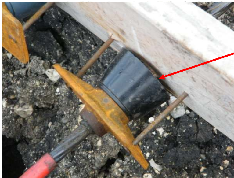
FIG. 2 ANCHOR ATTACHMENT TO FORMS
