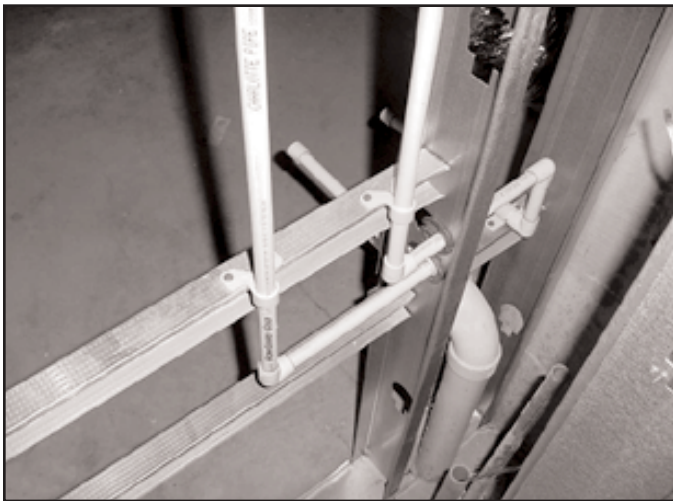
FlowGuard Gold® pipe support at metal studs.
