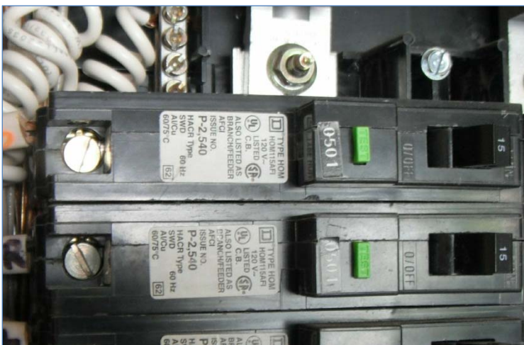
Figure 2 Branch/Feeder AFCI Label
